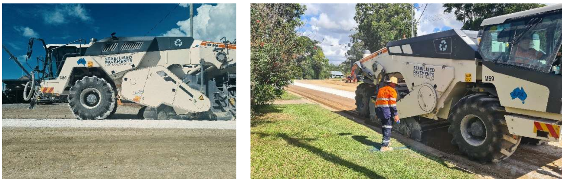
Figure 17: Mixing 60/40 Slag/Lime
