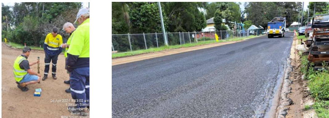
Figure 19: Bitumen Sealing
