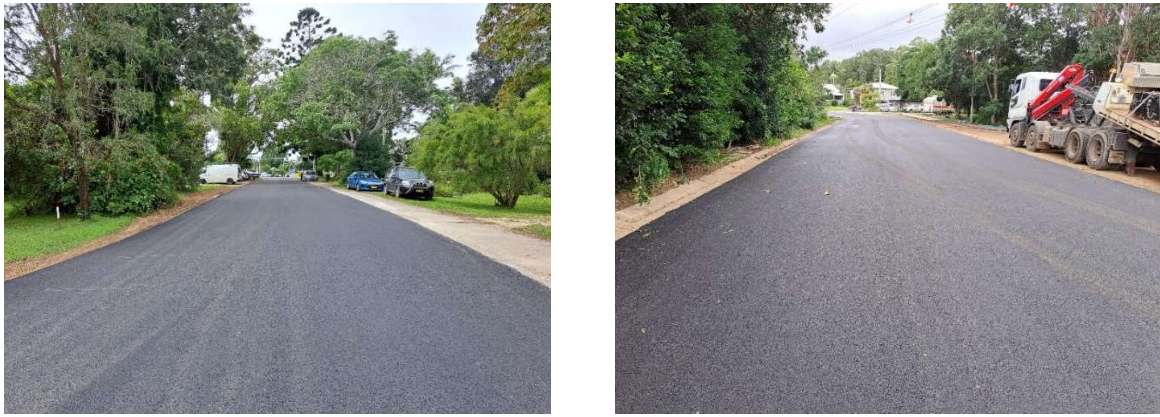
Figure 20: Post Asphalt Placement (01 May 2024)
