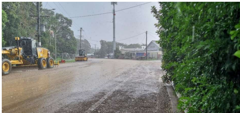
Figure 18: Wet Weather Prior to Sealing
