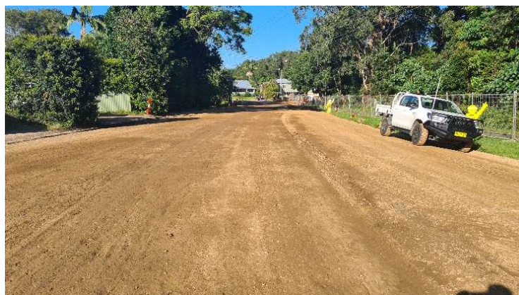
Figure 15: Lime Treated Pavement during Amelioration Period
