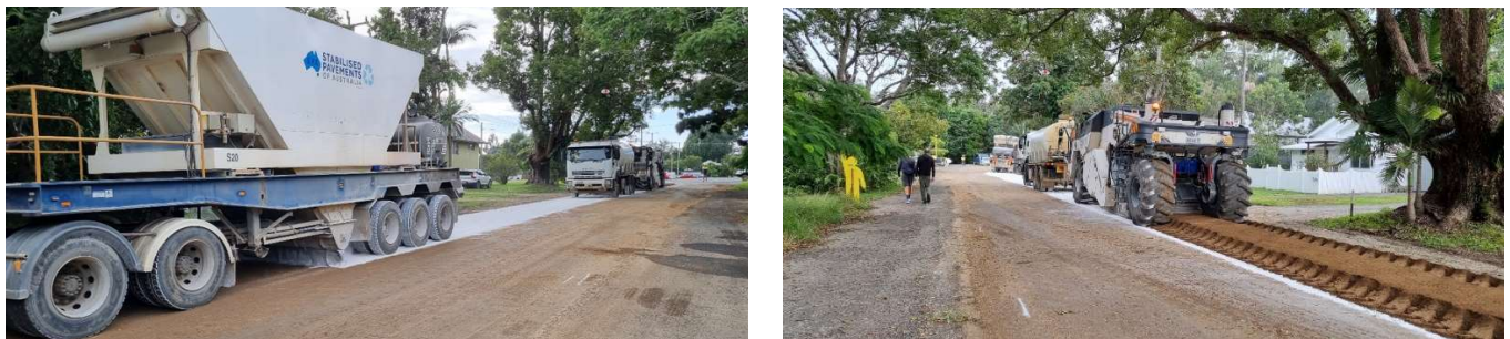
Figure 14: Spreading and Mixing Lime
