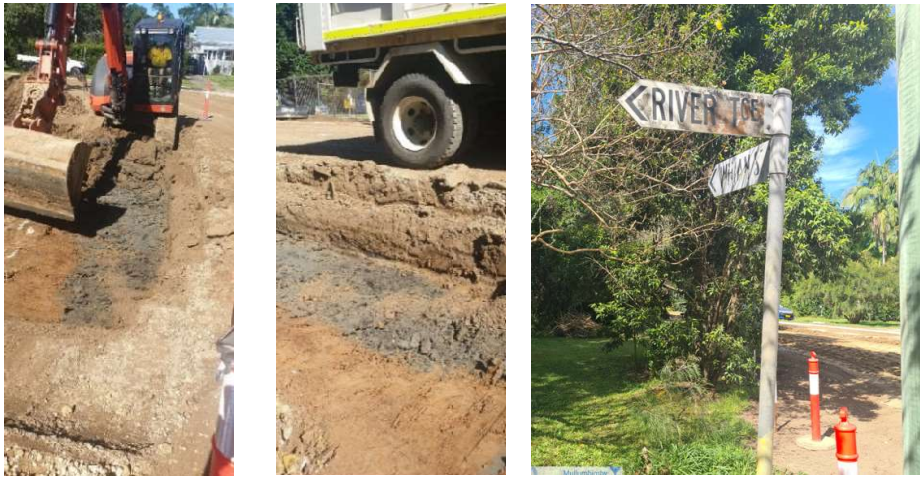
Figure 16: Soft Subgrade Repair
