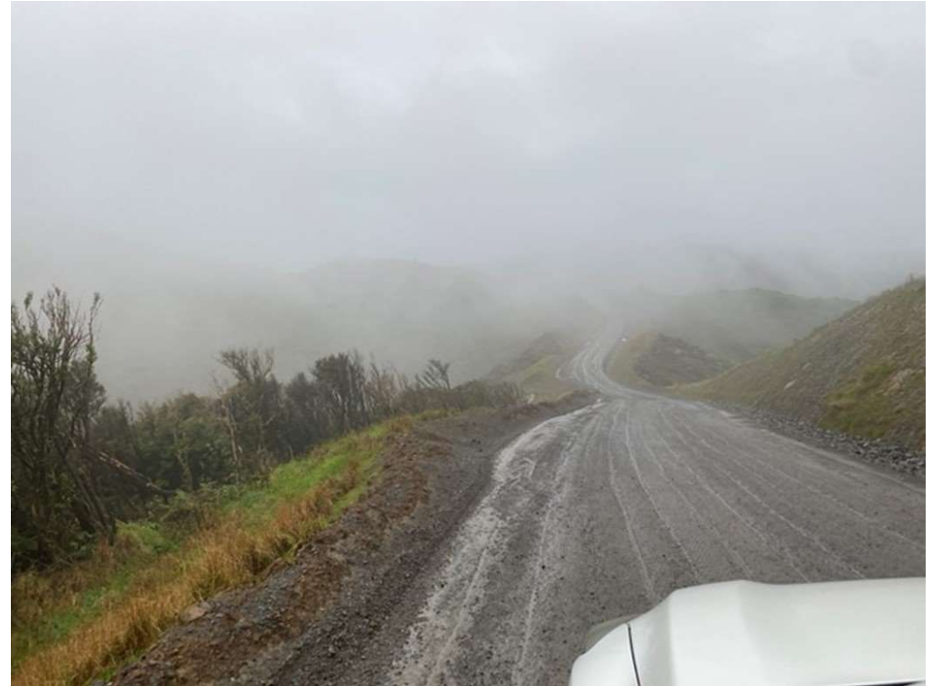
CTB Treated Access Track – Grades >15%
