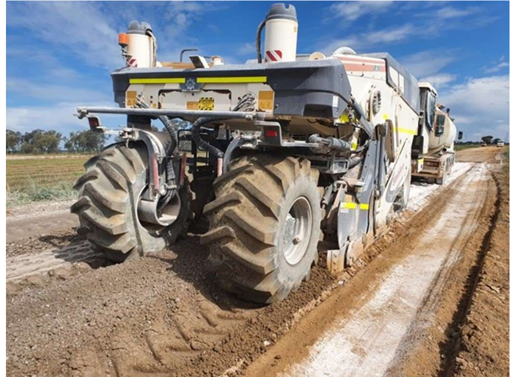
Lime Application - Mixing
