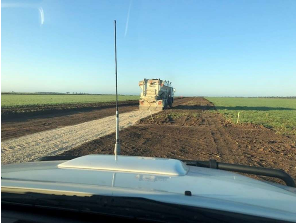
Lime Application – Spreading over access track
