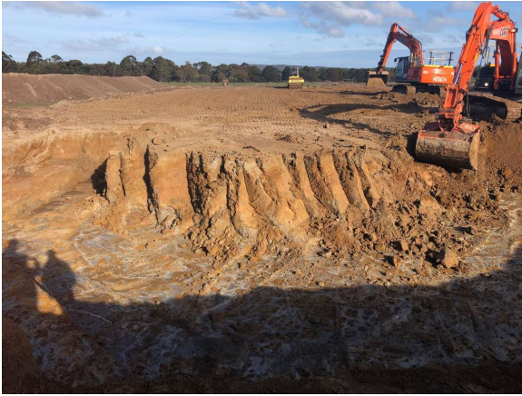
Source: icubed, Footing Excavation Lal Lal Wind Farm, 2019
