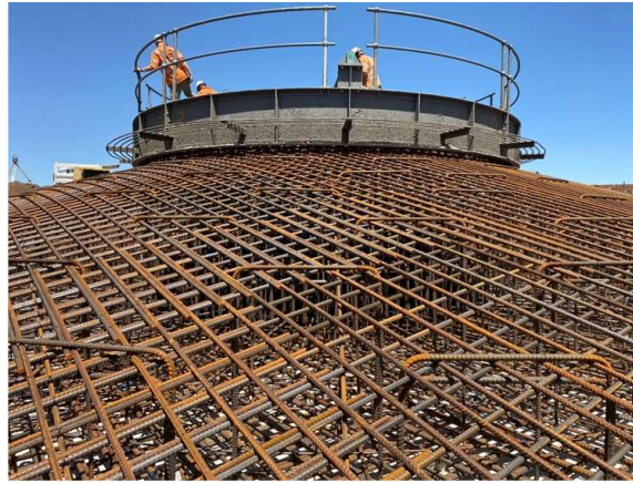
Source: icubed, Footing Excavation Lal Lal Wind Farm, 2019
