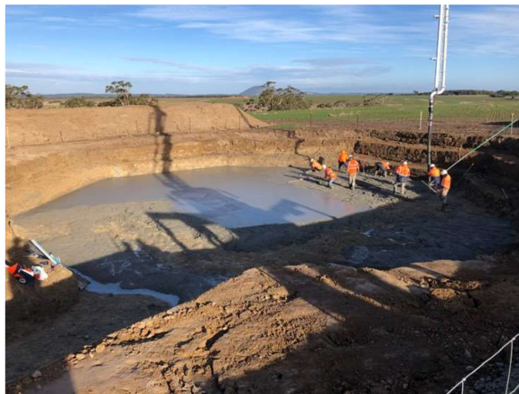
Source: icubed, Blinding Concrete Pour, Lal Lal Wind Farm, 2019
