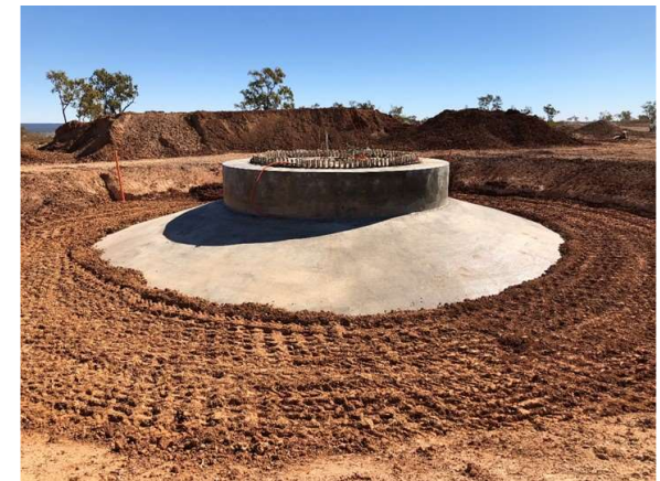
Source: icubed, Partially Backfilled Footing, Kennedy Energy Park, 2018
