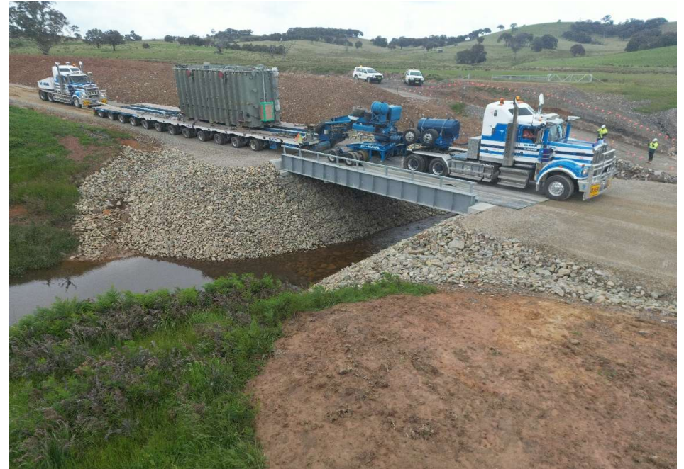
Transformer Delivery Vehicle
