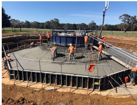
Source: icubed, Concrete Pour, Lal Lal Wind Farm, 2019
