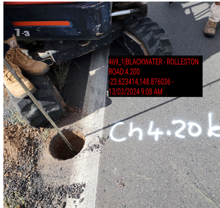
Prior to construction
