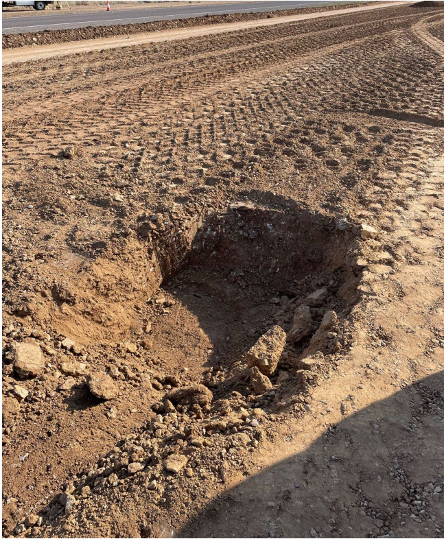
Test density in lowest 150mm
