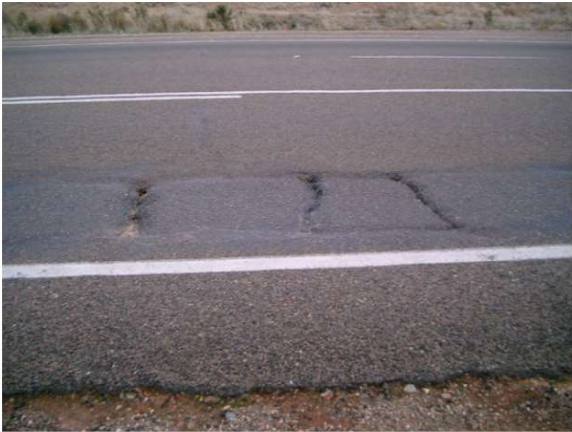
Figure 2.2: A fatigued cemented base pavement showing block cracking on a highway pavement in South Australia
