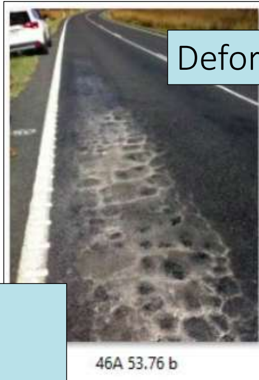
Figure 2.2: A fatigued cemented base pavement showing block cracking on a highway pavement in South Australia
