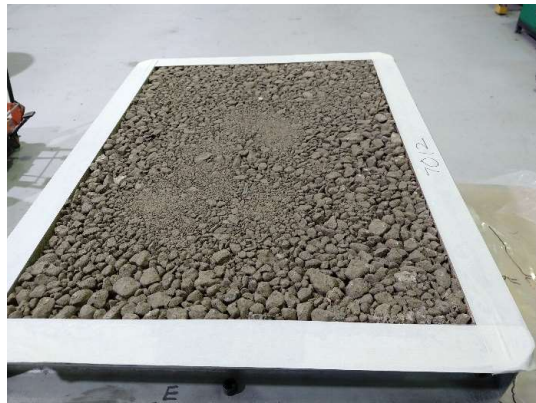
Surface after compaction
