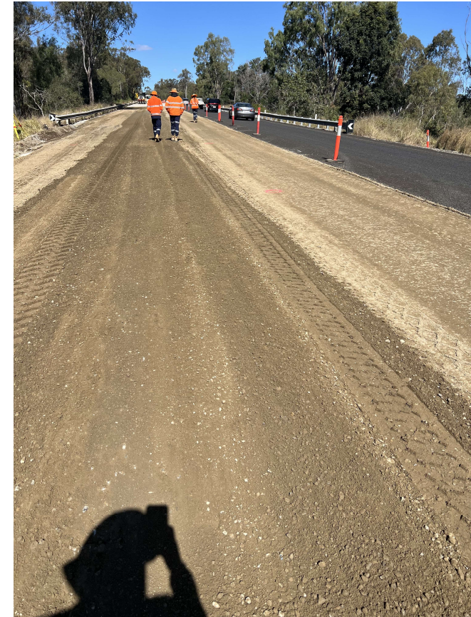
Start of Final compaction with smooth drum
