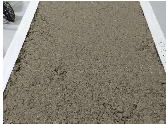
Surface after compaction
