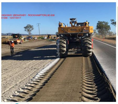
Triple blend improves the subbases stiffness and load bearing capacity
