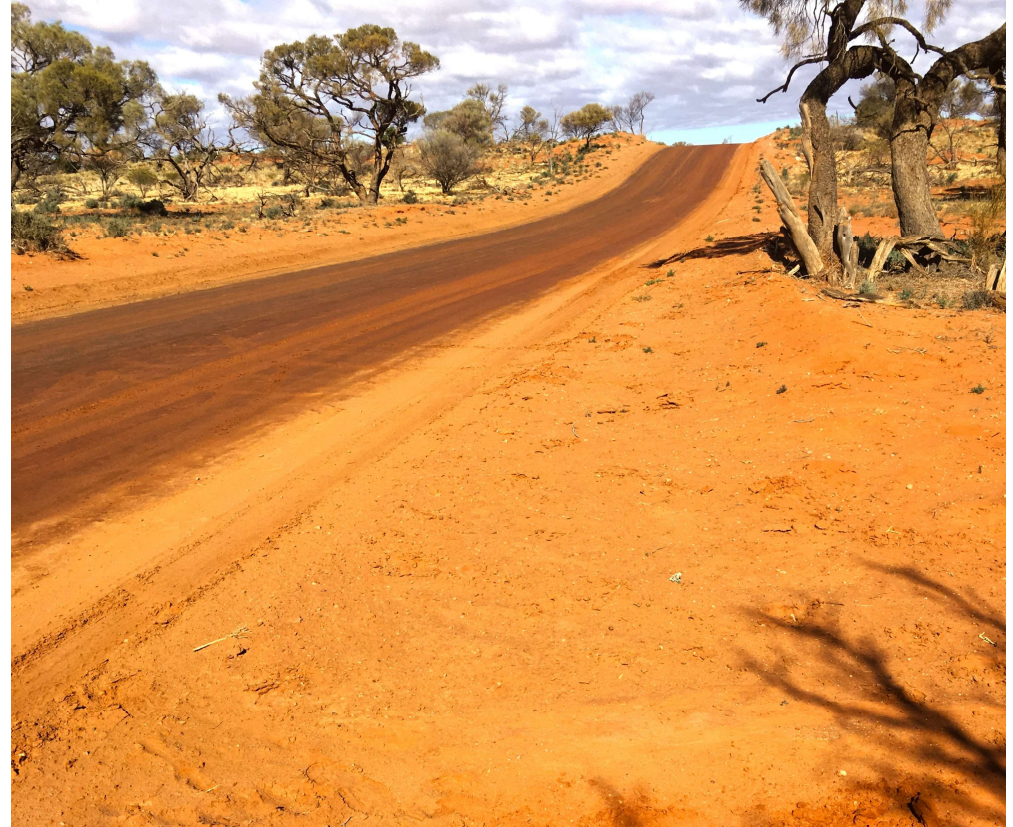
Carrapateena NBT and SAR Upgrades, SA Pavement Engineer
