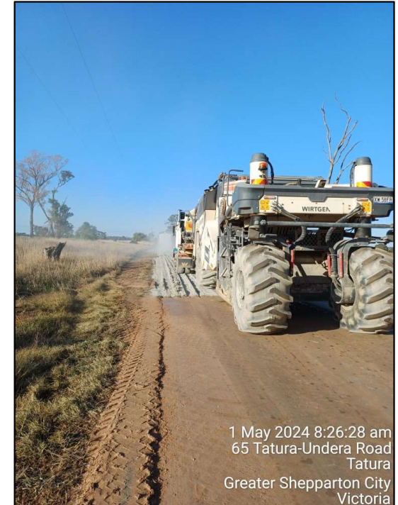
Figure 4: Stabilisation of In-situ Subgrade Material
