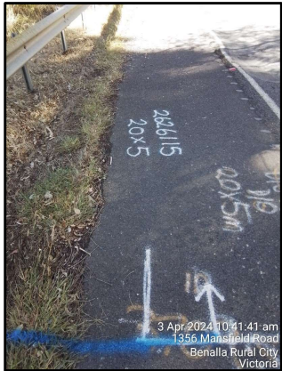
Figure 6: Scoping of Patch Locations prior to Commencement
