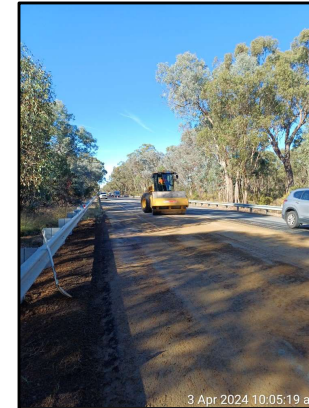
Figure 9: Compaction Effort on treated Subgrade Layer
