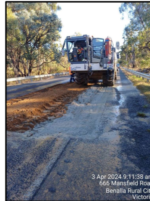
Figure 8: First run of Triple Blend Stabilising Completed
