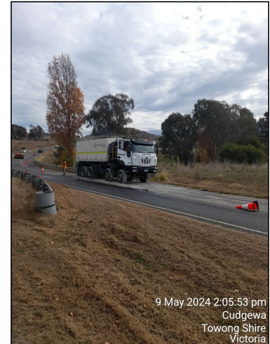
Figure 5: Stabilisation of In-situ Subgrade Material
