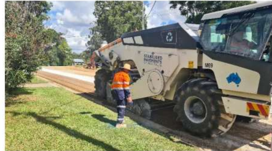
Figure 17: Mixing 60/40 Slag/Lime
