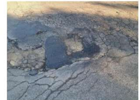
Figure 5: River Terrace Pavement Condition [2]
