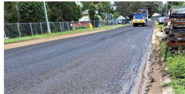
Figure 19: Bitumen Sealing
