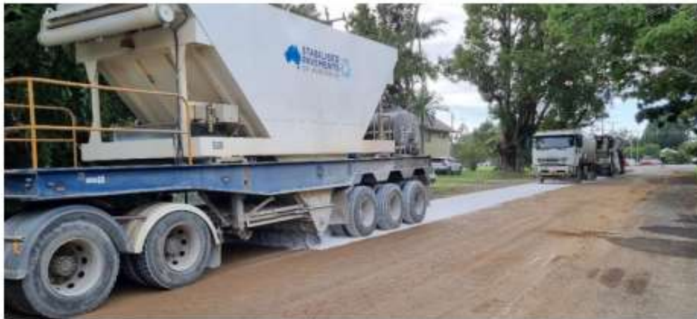
Figure 14: Spreading and Mixing Lime
