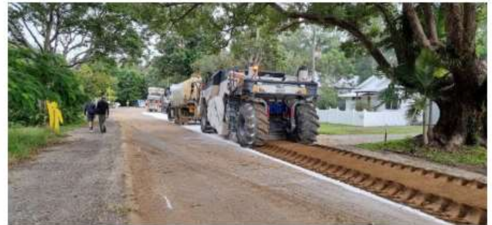
Figure 14: Spreading and Mixing Lime
