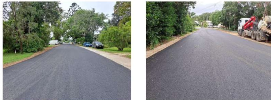
Figure 20: Post Asphalt Placement (01 May 2024)
