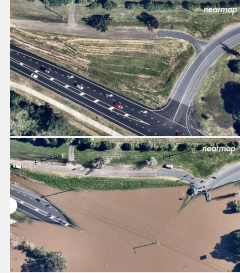
NSW – N. England Hwy July 2022
