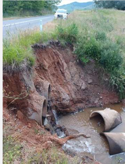
Culvert failures
