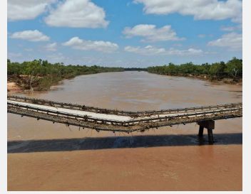
WA - Fitzroy River Bridge December 2022
