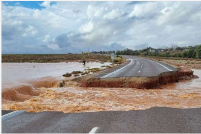
SA – Olympic Dam Hwy January 2022
