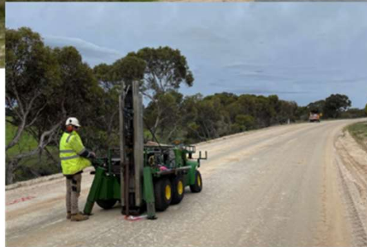
Geotechnical Investigation – Unsealed Section to be upgraded
