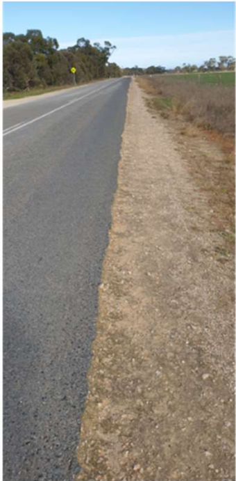
Typical - Unsealed Shoulder Pavement widening and shoulder construction
