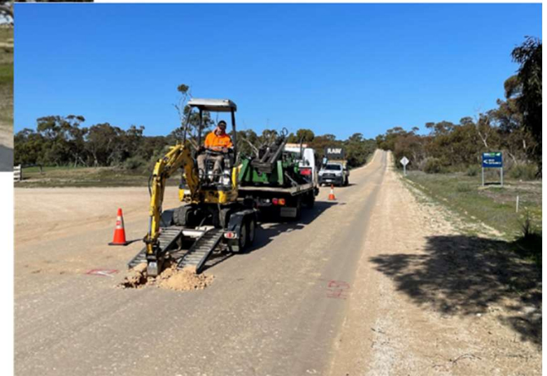
Test Pit – Unsealed Section to be Upgraded
