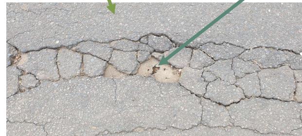
Crocodile Cracking
