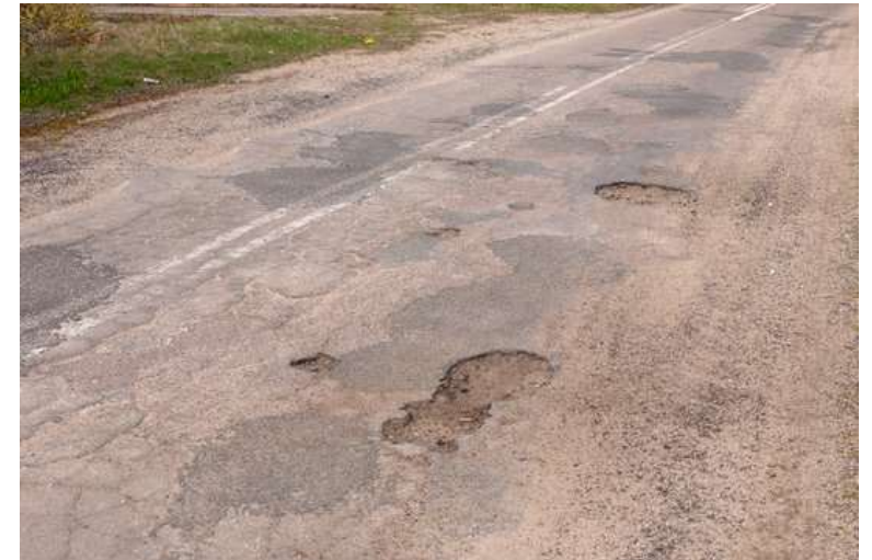
Example rural pavement (Google 2022)
