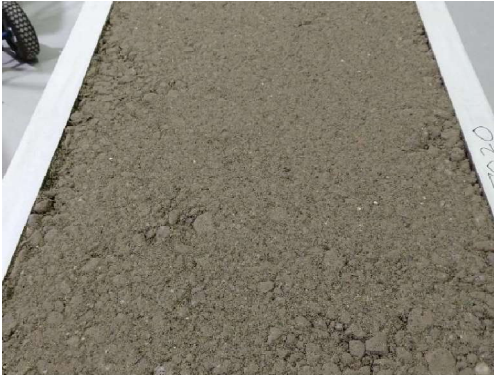
Surface after compaction
