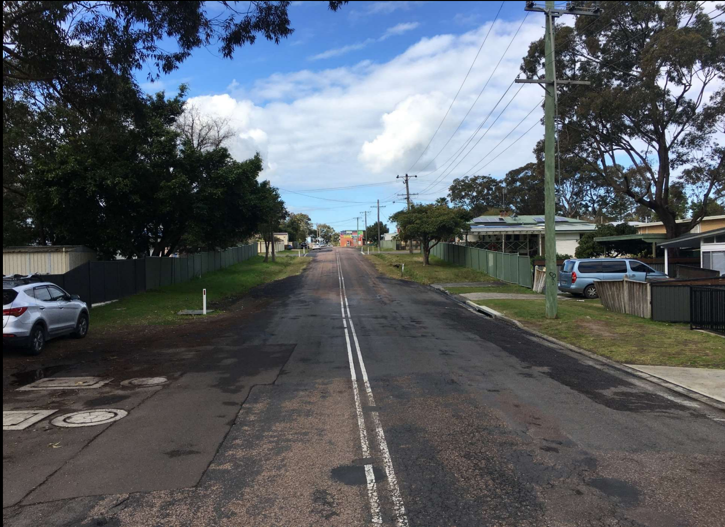
Road Construction – Utilising Recycled Products
