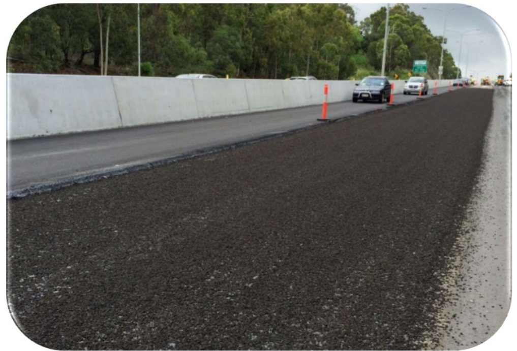
Smith Street Motorway 2015 – Eastbound
