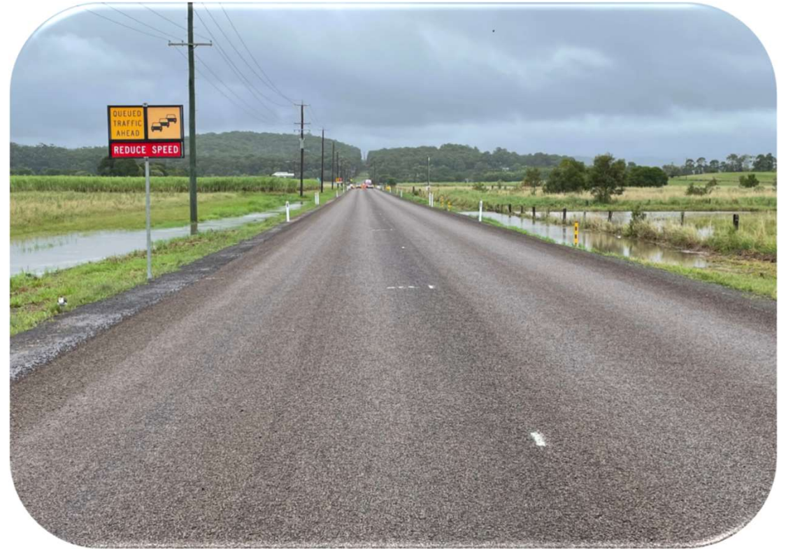
After flooding foamed bitumen treated section
