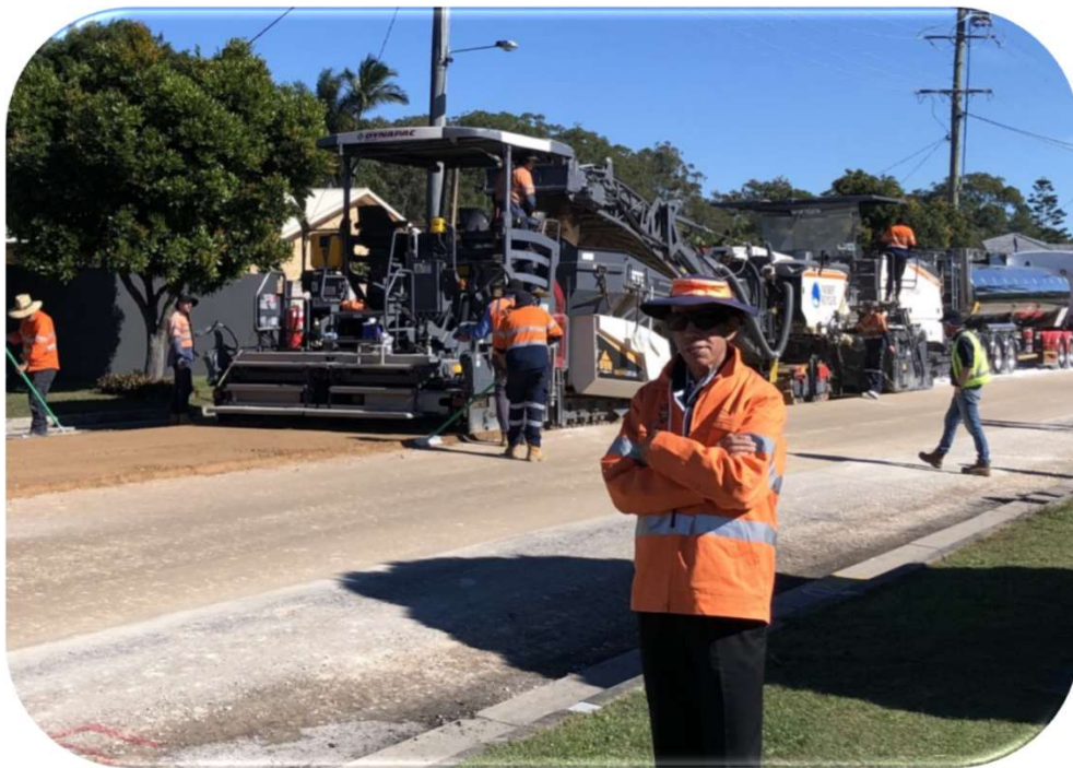
W 380 CR (Paver Laid Insitu Foamed Bitumen)
