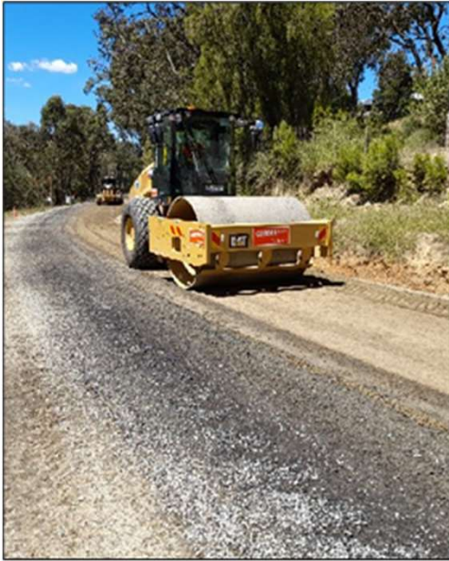
Figure 8: Compaction Effort on treated Subgrade Layer
