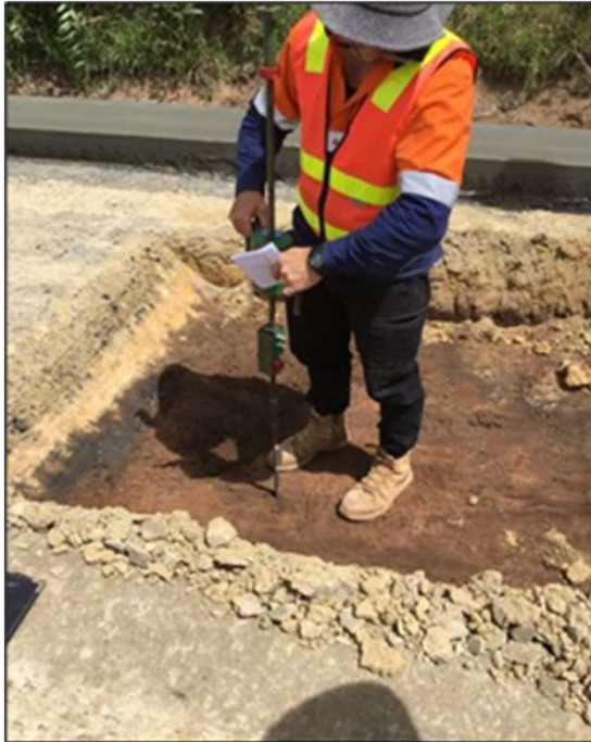
Figure 5: DCP Testing on Lower Subgrade Layer
