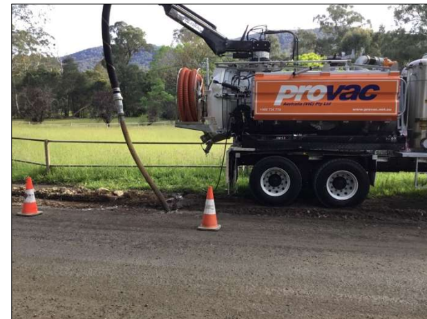
Figure 3: Locating Underground Services within pavement construction envelope
