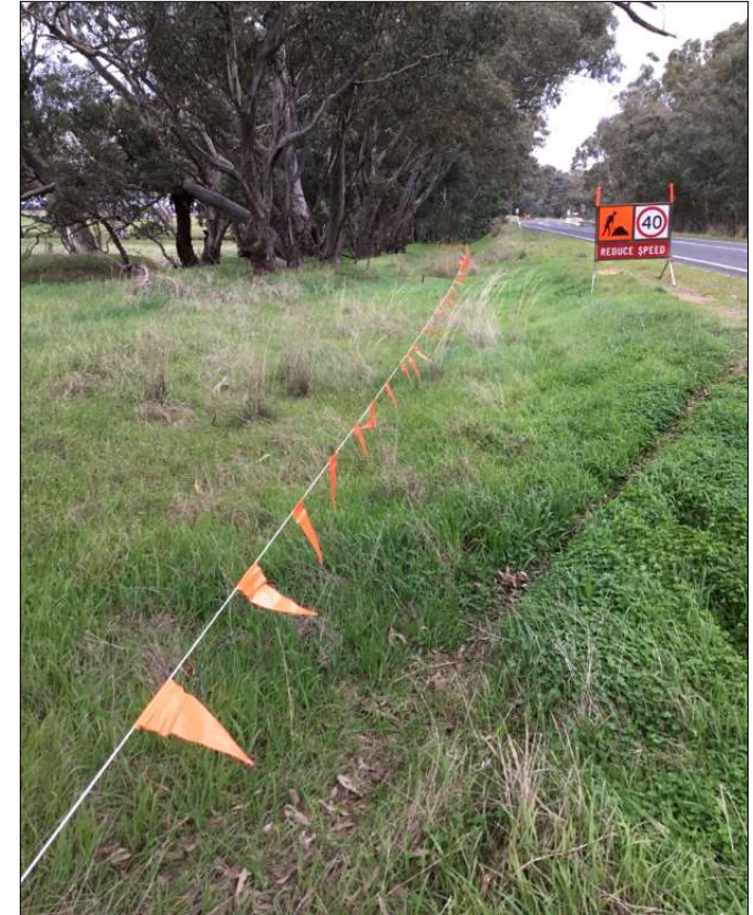
Figure 4: No Go Zone Fencing Installed
