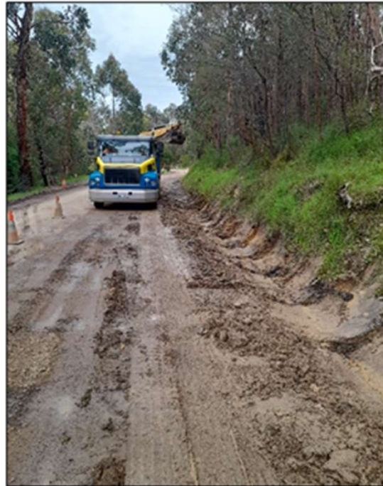
Figure 6: Struggling to keep the Subgrade Trafficable
