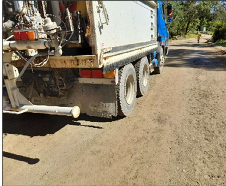
Figure 9: Proof Roll of Subgrade Layer & ITP Sign off with VicRoads
