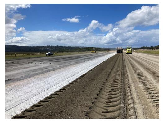
"The entire existing pavement and seal was able to be reused in the recycled pavement at Merimbula Airport, which meant that only a minimal amount of material had to be imported to build the pavement to the new levels. Trimmings from the pavement re-shaping works were used to build a new runway shoulder and any excess material was reused in the new taxiways being constructed." – Alex Warren, Project Engineer, Symal Infrastructure
