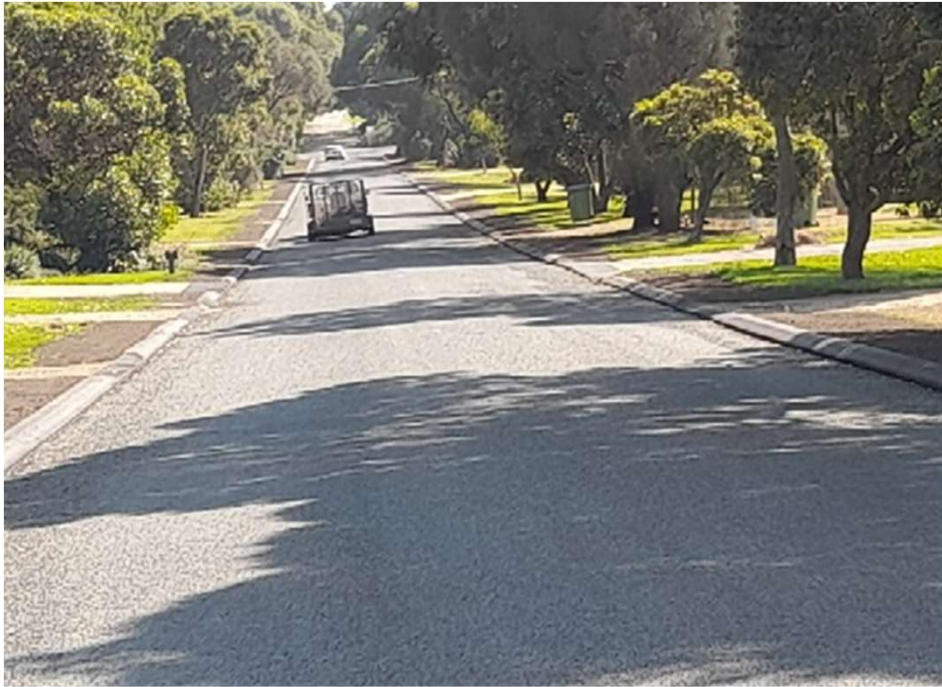
Finished road being used by locals
