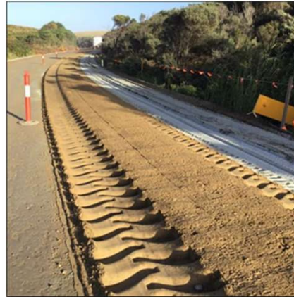
First run of cement stabilising completed
