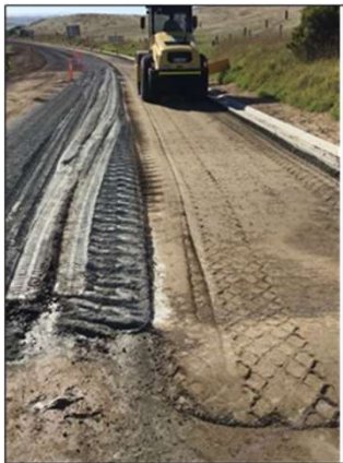
Compaction effort on treated subgrade layer
