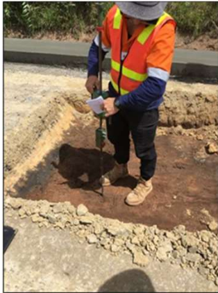
DCP testing on lower subgrade layer
