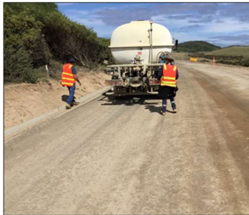
Proof roll of subgrade layer and ITP sign-off with VicRoads
