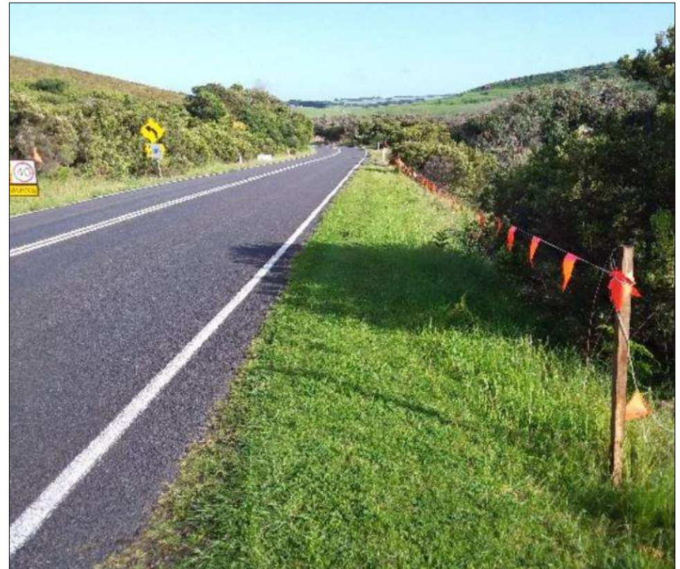
No Go Zone fencing installed
