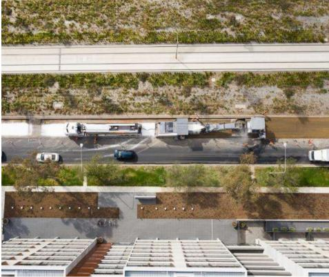
Paver-laid treated material had an initial compaction upon placement and controlled levels, eliminating the need of a grader and requiring only one roller for final compaction
