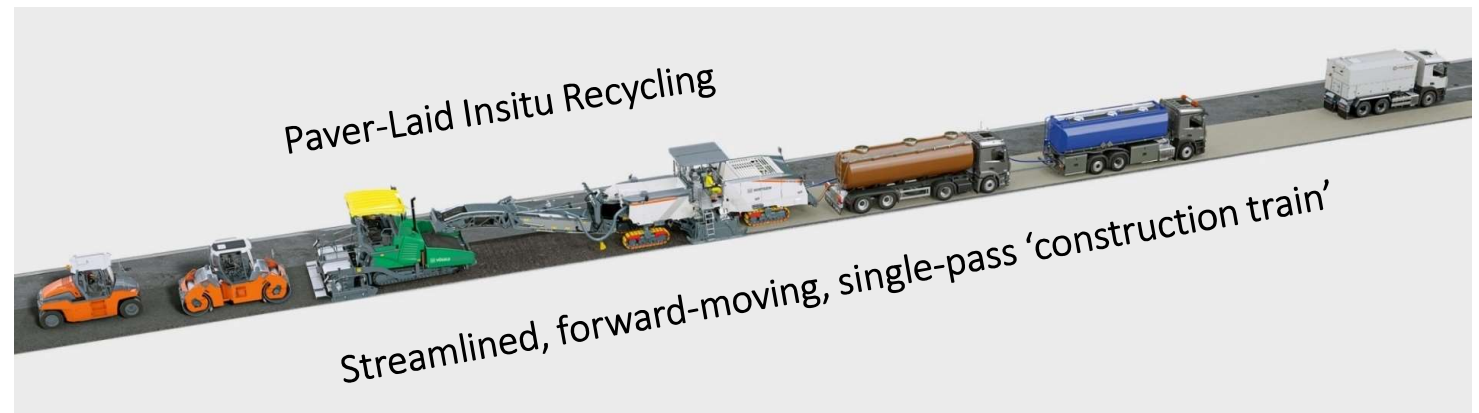
Visual of the W380CR and the full construction train, which is forward-moving without reversing
