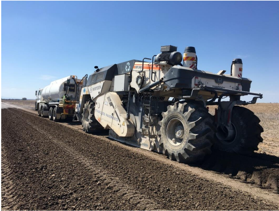
Mixing and moisture conditioning.
