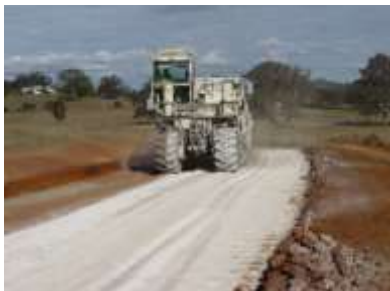
Figure 1. Lime Stabilisation of Subgrade Materials
