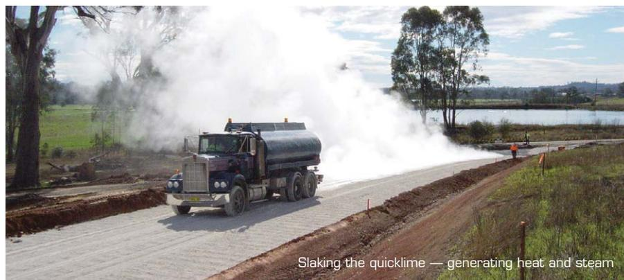
Slaking the quicklime — generating heat and steam
