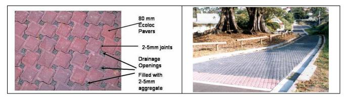
Figure 8 Permeable concrete eco-paving using concrete segmental pavers.
