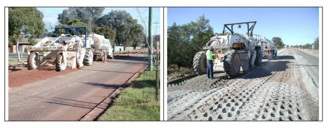
Figure 2 DPP being used in urban and rural sites using conventional insitu stabilisation equipment.
