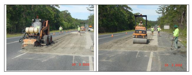
Figure 3 View of skidsteer and smooth drum roller system for small pavement patch repairs.
