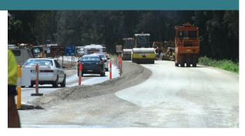
As this is a new research area for RMS, the *Austroad's Guide to Pavement Technology* principles was applied to the project, which was designed as a continuously bound layer, with the expected modes of distress being rutting and/or shoving due to insufficient resistance to pavement deformation and cracking due to fatigue.
