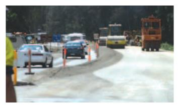
NSW RMS - Farlow's Flat - Plant mixed Foamed Bitumen stabilisation works completed under traffic
