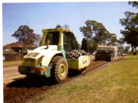
Foamed Bitumen Stabilisation Cumberland Highway Campbelltown - One of Campbelltown City Council's 261 stabilisation jobs since 1991
