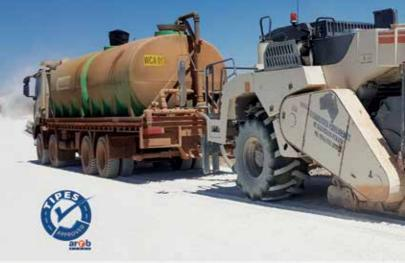
Polyroad is an extremely useful stabilisation binder, enabling us to extend the range of materials suitable for stabilisation, and thereby conserve a greater quantity of natural materials. Being a dry powder polymer ( DPP ) Polyroad is insoluble in water and most importantly does not degrade or leech in the field. When stabilising with Polyroad
