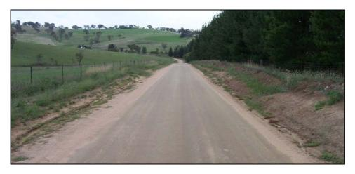
Figure 2 Unsealed road stabilised with lime to suppress dust generation and provide stiffness to carry heavy traffic loads.
