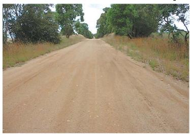
Above: Two year old stabilised pavement which has no maintenance.
