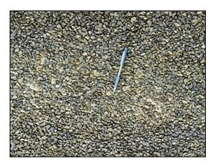
*Figure 5* View of stabilised pavement with 7 mm crushed aggregate on surface.
