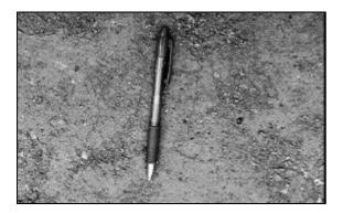
Figure 3 Fine micro-cracks develop on the surface in a stabilised layer, but pose no detrimental problems.
