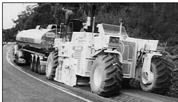
Figure 6 View of tanker in front of stabiliser/reclaimer during mixing operation.
